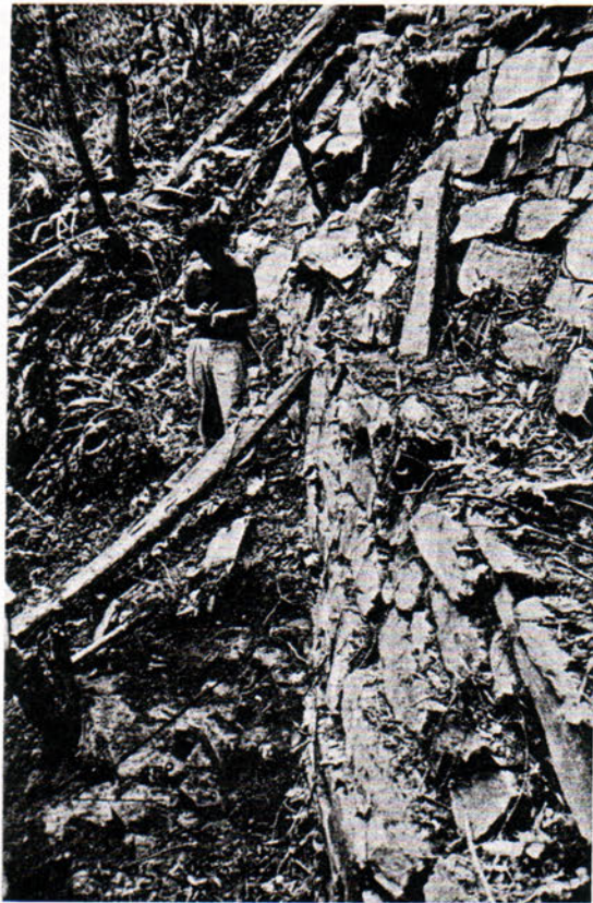
Foundation Stone Wall
